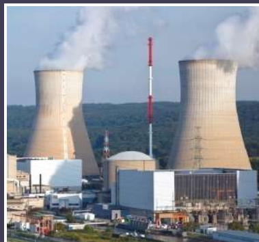
Thermal Power Plants
